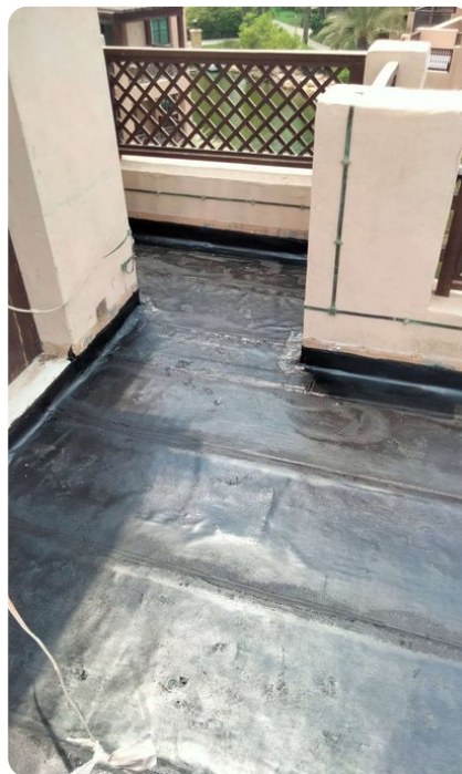
Membrane at terrace & parapets
