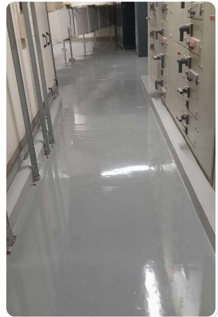
3. Application of 2-3mm epoxy
