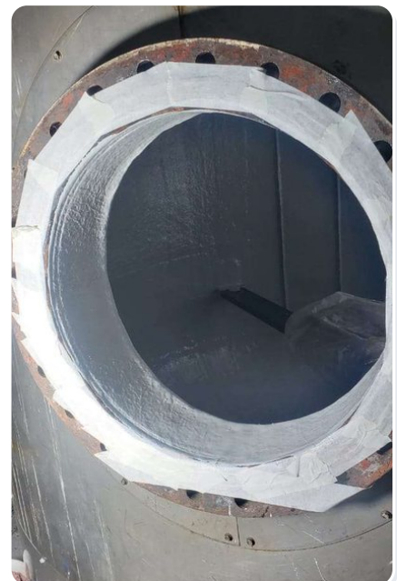
Manhole & access opening
