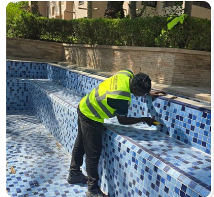
Grouting at pool wall
