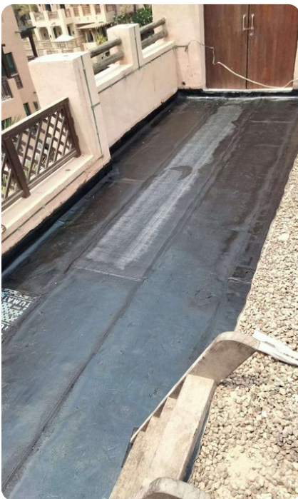
Torch-applied membrane
