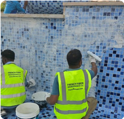
Epoxy grout applied to wall tiles
