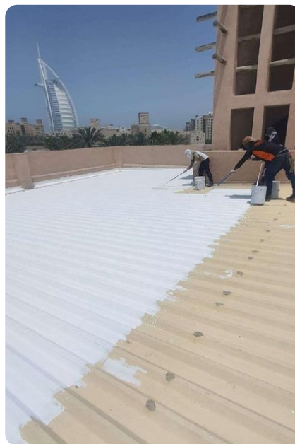
Cross-directional coating in progress
