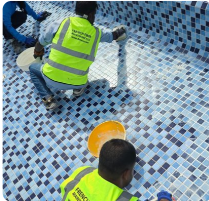
Epoxy grouting of floor tiles
