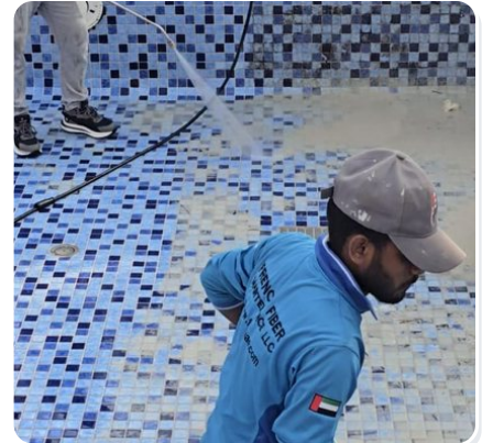
Surface brushing & rinsing
