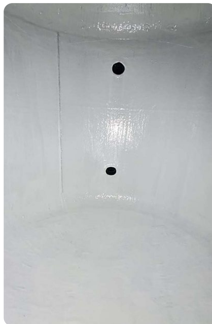
Finished interior coating
