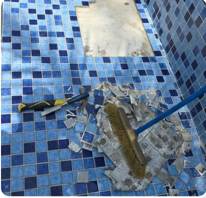
Removing deteriorated grout
