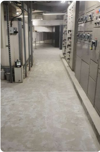
1. Floor grinding
