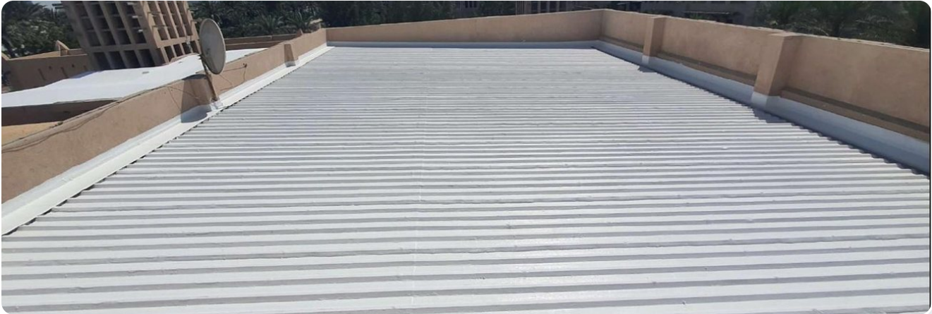
Completed roof coating
