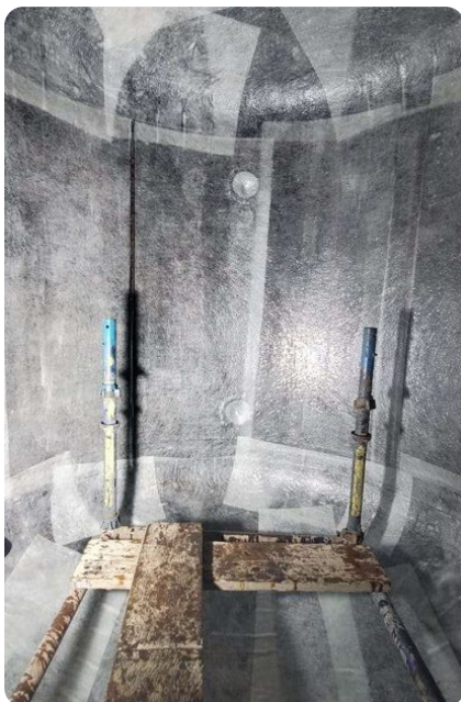
Tank interior – lining works
