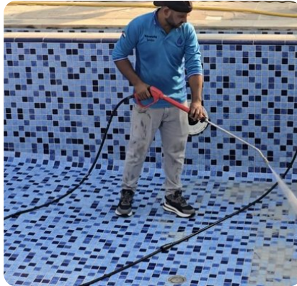
Pressure washing of the basin
