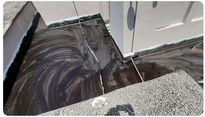
Priming at roof upstands
